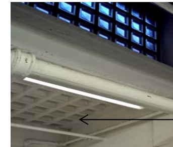
Existing pavement lights along Drummond St
