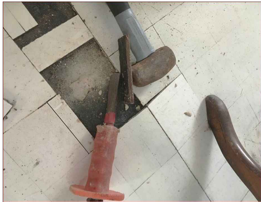
Image of the structure of the Existing flooring
