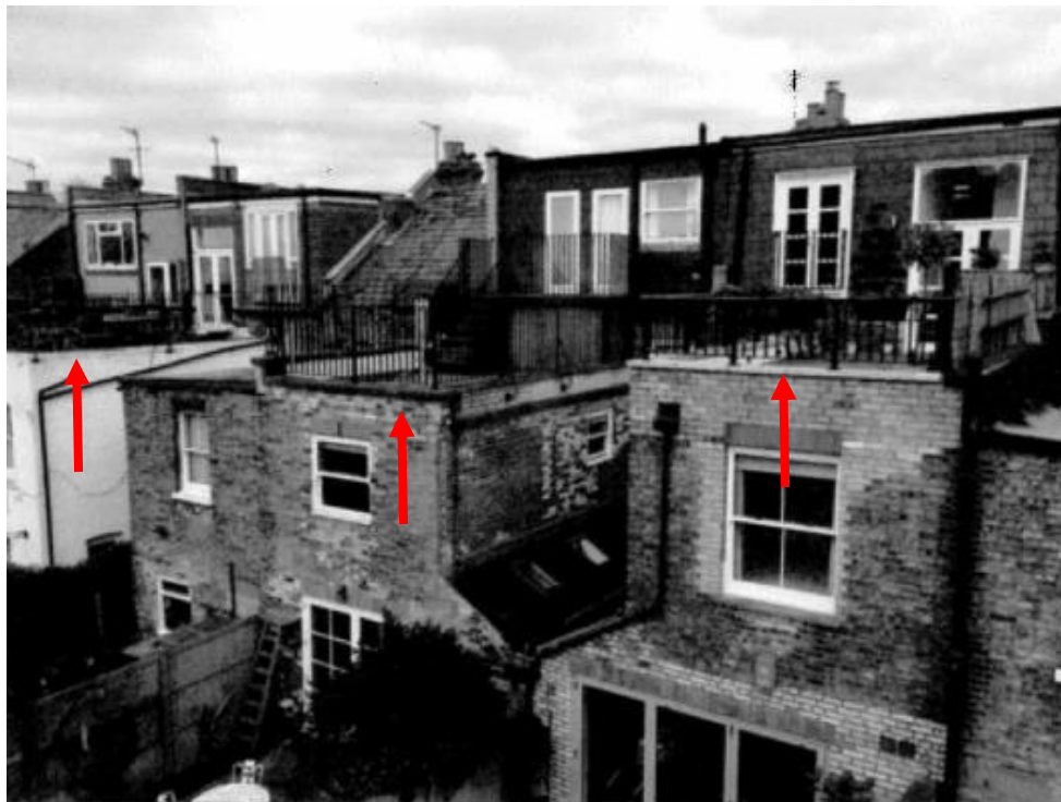
Plate 4. View taken from No.47 Burrard Road showing roof terraces at Nos. 7, 9 & 13 Ingham Road.
