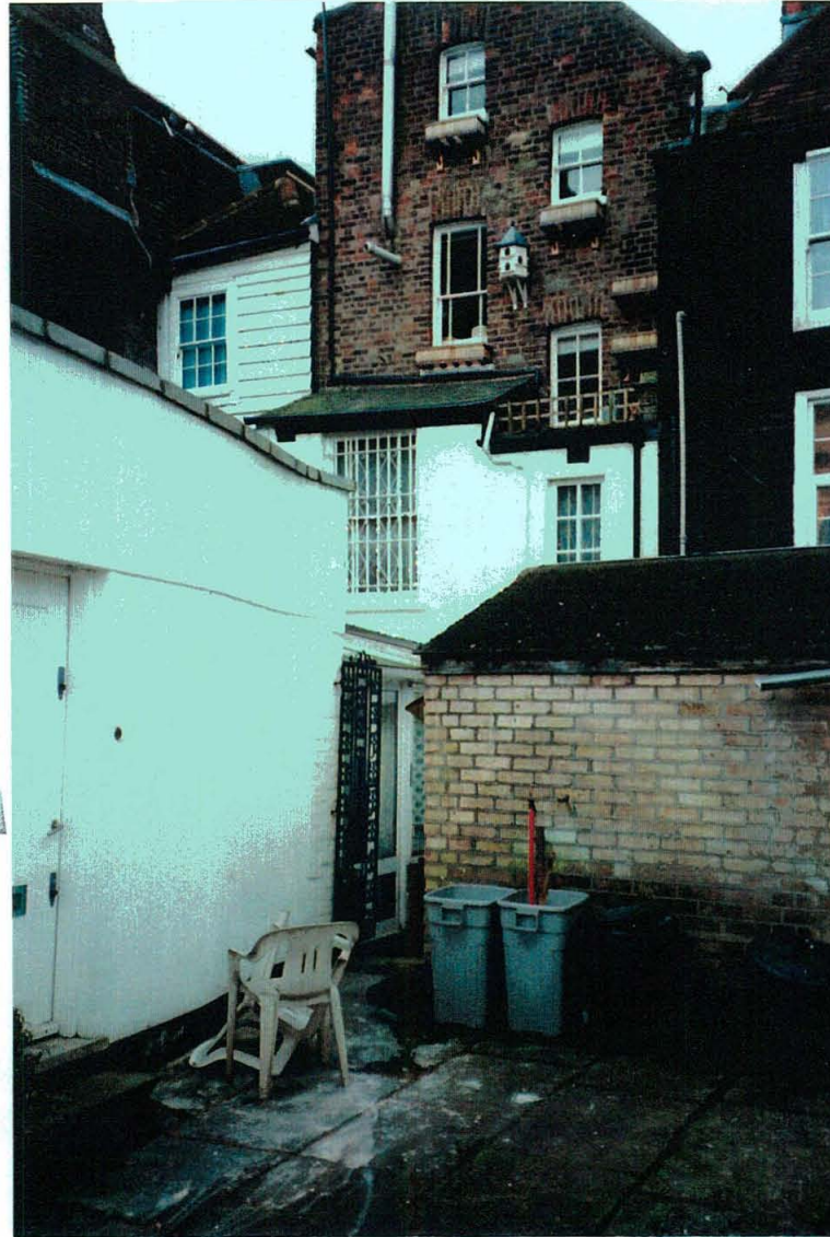
view of rear of property
