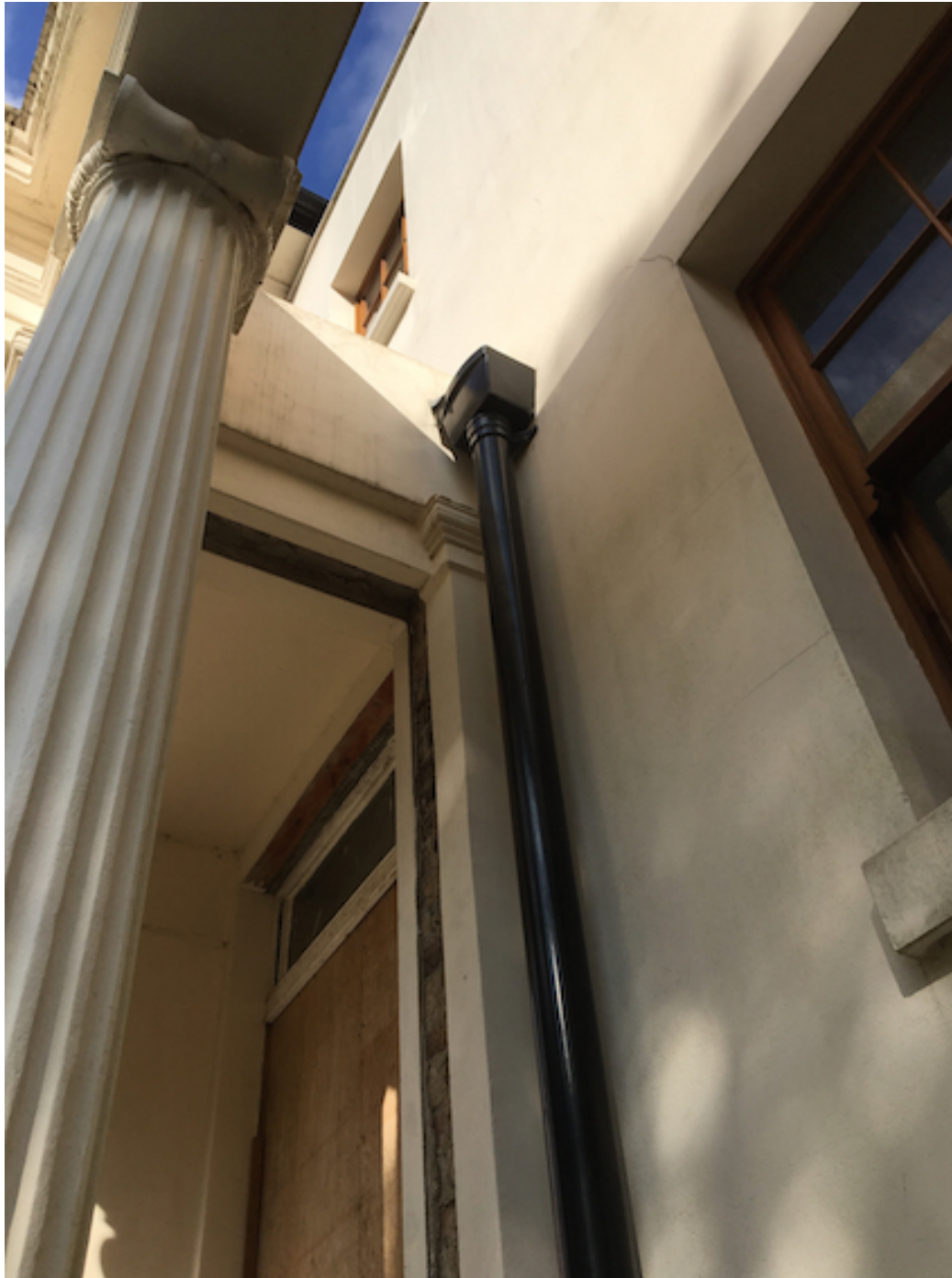
Photo.4 Example of the as installed rainwater pipework due for replacement. (Oct 2016)
