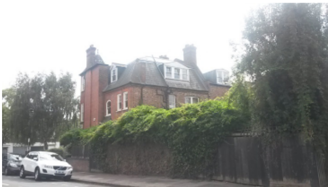
Photo 8 (above): View of side and rear elevations of No. 59 Croftdown Road, looking south from Brookfield Park
