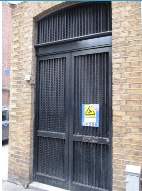
Example of Existing Substation Door
