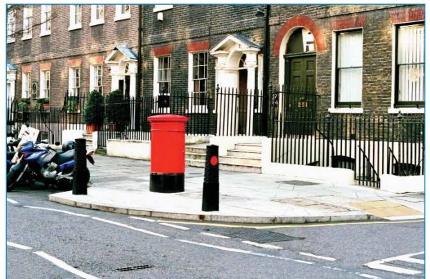
Footway build-out in John Street
