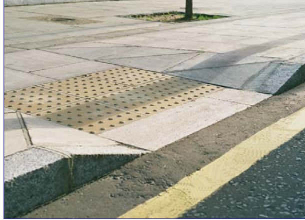
Details of dropped kerbing in John St
