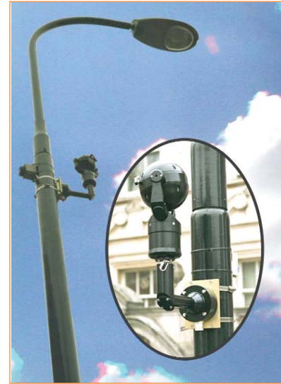
‘Metal Mickie’ camera on a lighting column
