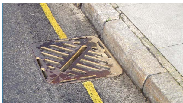
Carriageway gully cover – Double triangular D400
