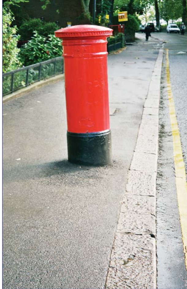
New bituminous footway on Regent's Park Road
