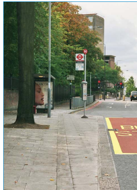
Obtuse bus boarder in Adelaide Road
