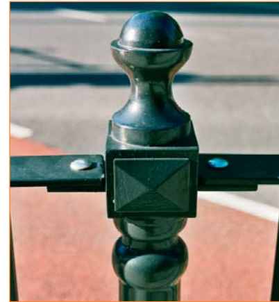
Detail of Folkestone guardrail
