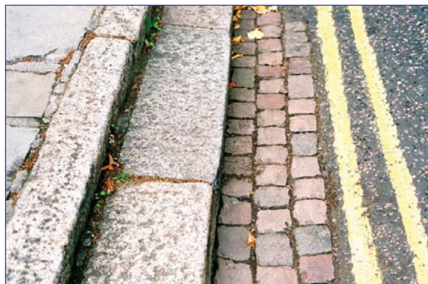
Double granite kerb with drainage channel
