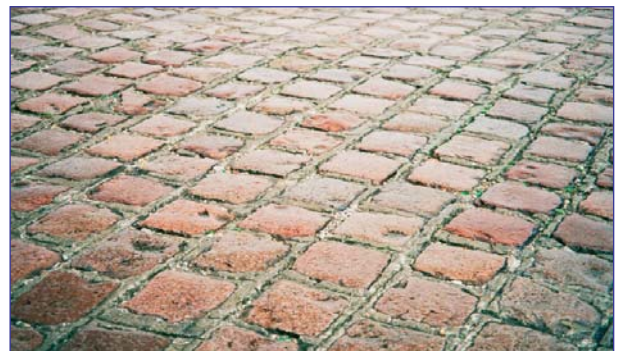
Old granite setts in Daleham Mews
