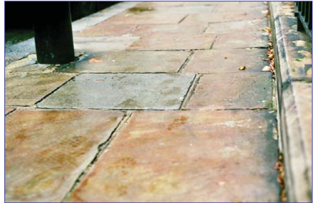
Old York stone re-laid with flush pointing
