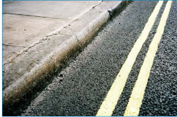
Primrose yellow lines at 50mm width
