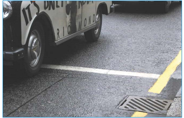
Carriageway in Marchmont Street
