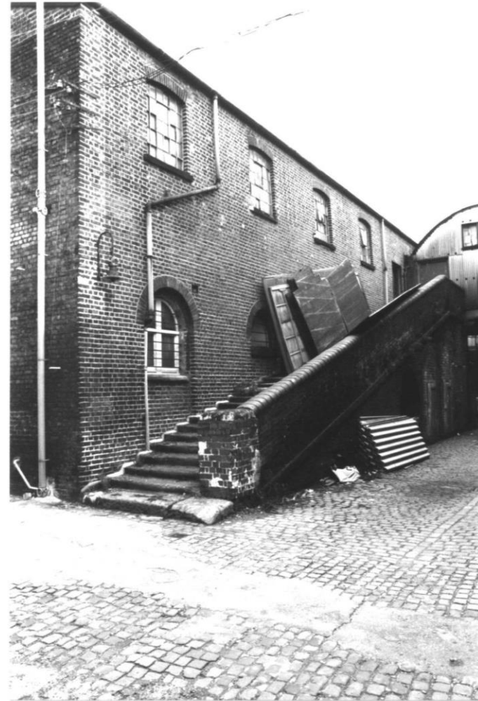
View South to bridge between Provender store (left) and Tack room
