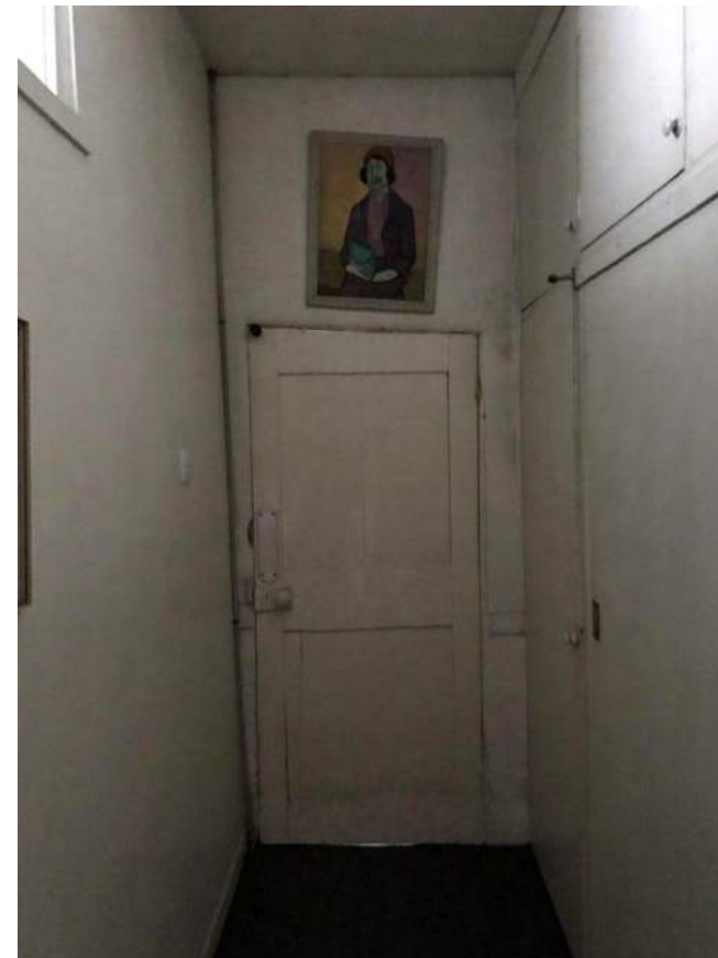
No architraves to first floor rear bedroom door
