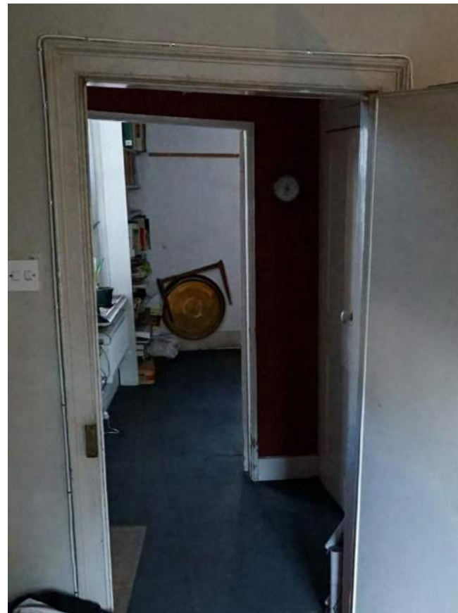
Non-original moulding added to sitting room architraves
