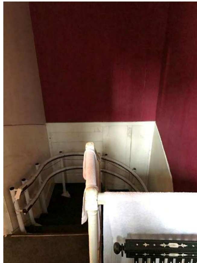
Non-original timber panelling to staircase to be replaced
