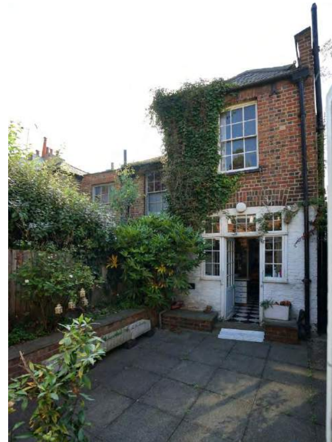
Existing first floor window to be retained. New windows to replace existing ground floor door and windows
