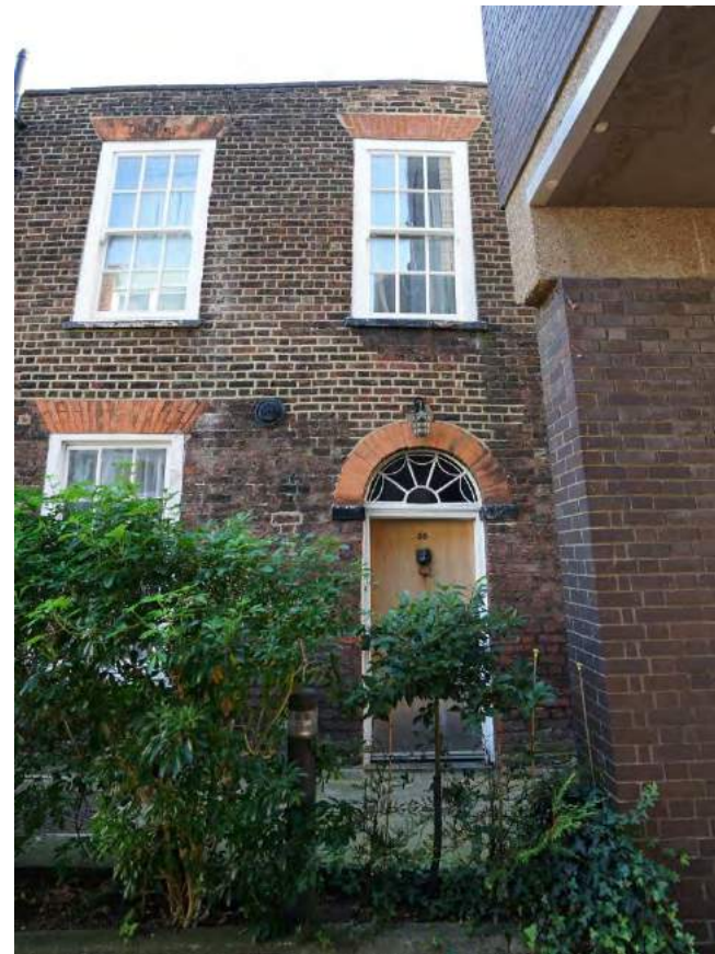
Non-original double glazed units to first floor
