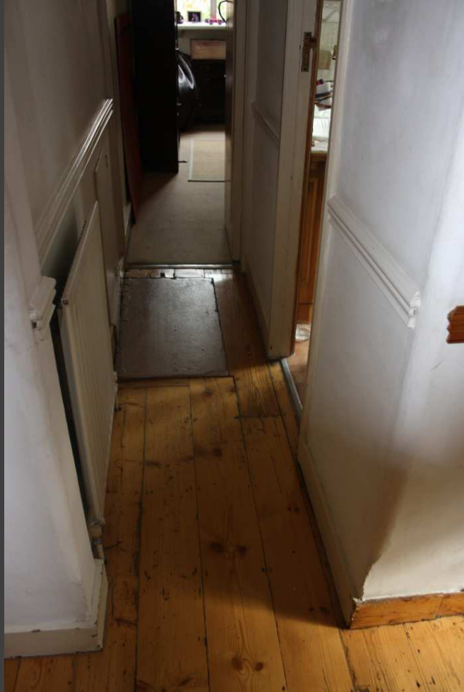
Views of bathroom partition at first floor level showing original hearth in floor.
