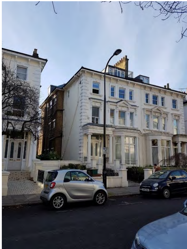
PS 11: Existing dormer at 19 E BPG (of smaller scale than 17 and 21 BPG)
