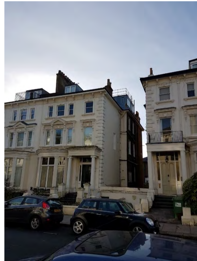
PS 12: The larger side dormer at 17 BPG (the “twin” to 19 E)
