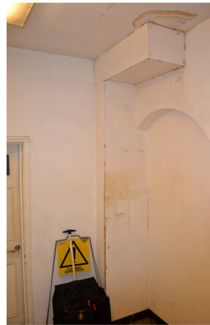
3 8MS/2/004 - Lobby (Riser carefully removed)
