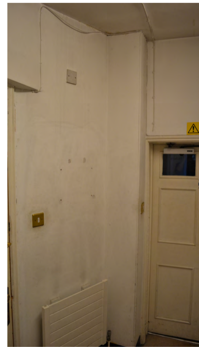
4 8MS/2/004 - Lobby (Riser carefully removed)
