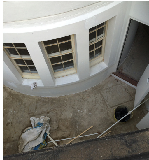
Typical light well as constructed
