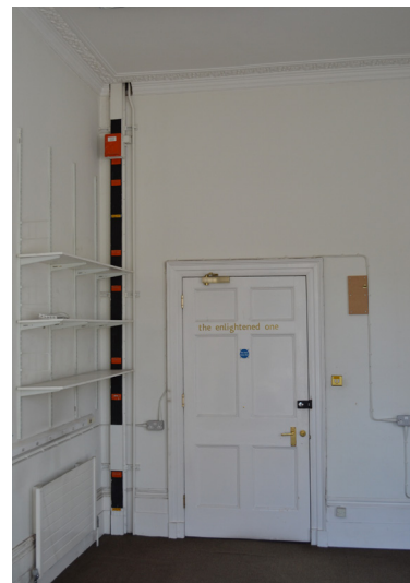
Typical existing riser location
