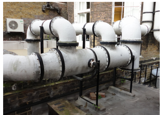
Typical rear elevation services pre- construction
