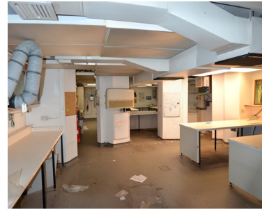
Typical basement image pre construction
