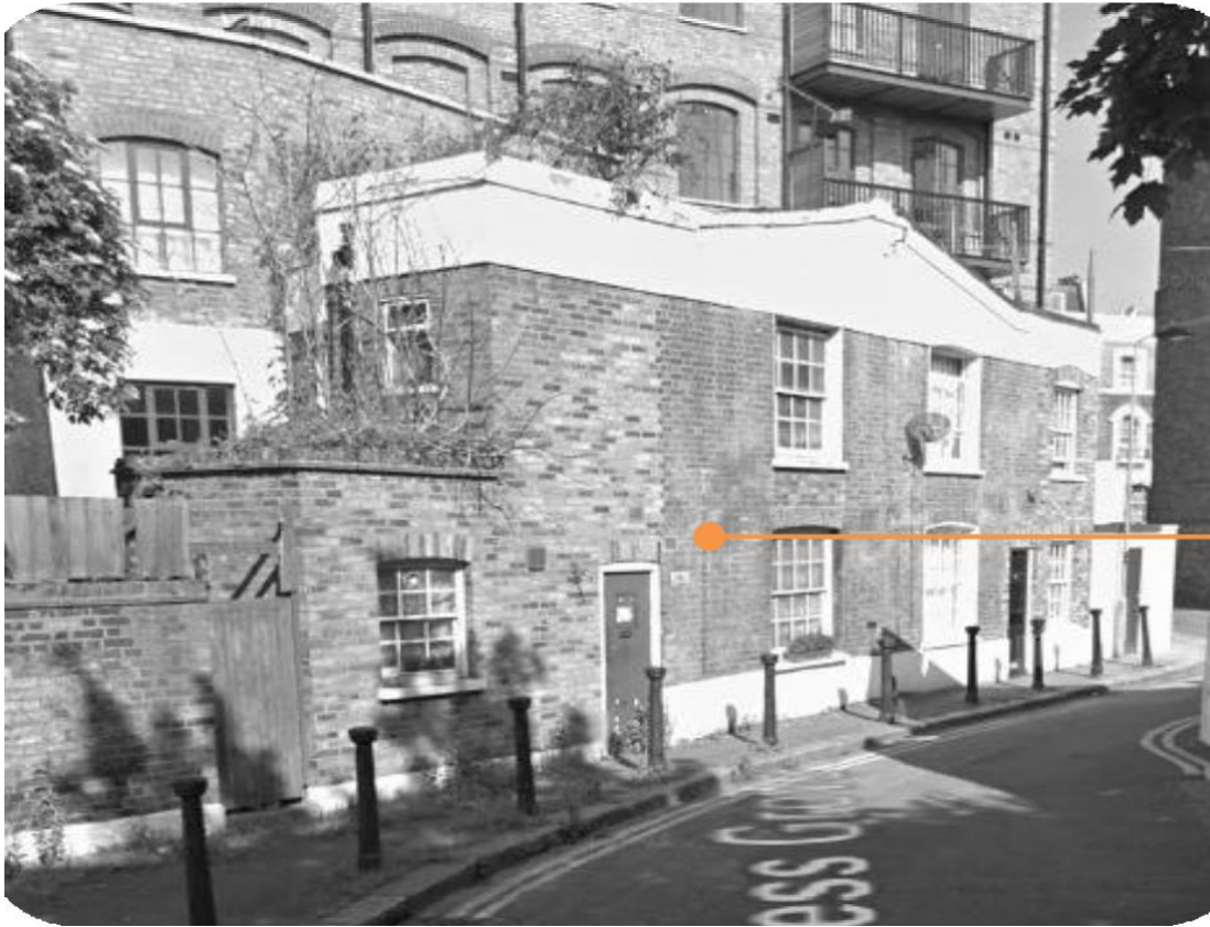
Image 1. Front elevation northwest elevation
