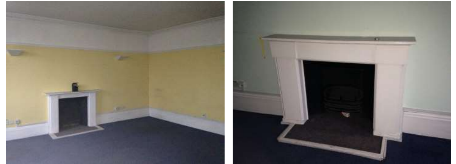
Figure 15: Office to the second floor, showing fireplace and surrounds with skirting, picture rails and cornicing.
