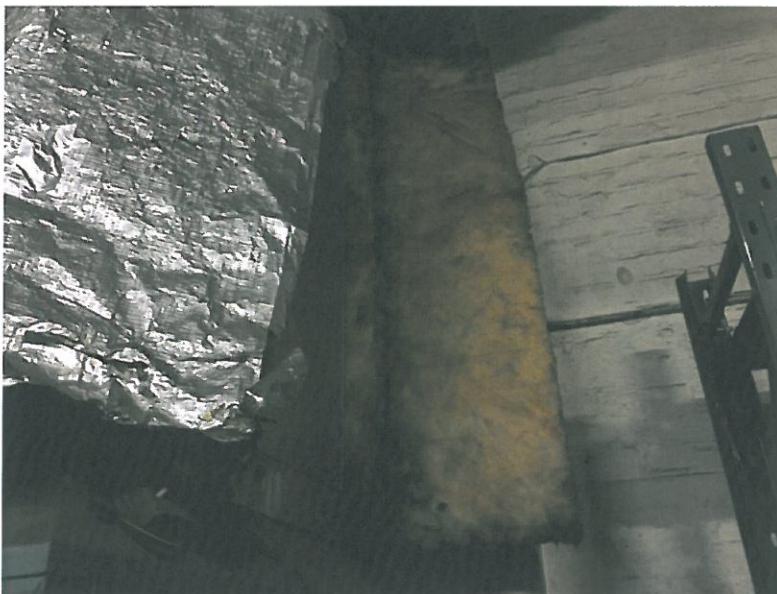
Sample 04 – Thermal insulation to heater unit – No asbestos detected.
