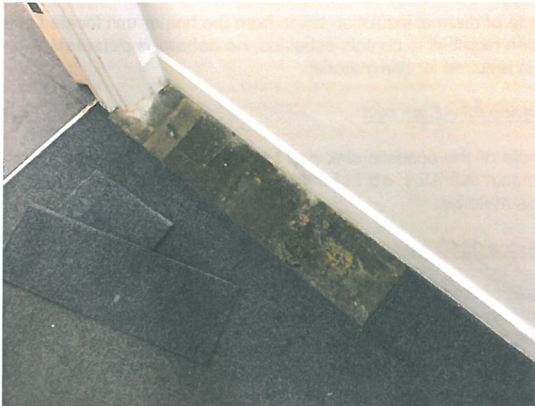
Sample 02 – Bitumen adhesive to floor – No asbestos detected.
