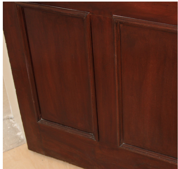
Finished door with sealmaster fireface membrane applied to flat mahogany door panels.
