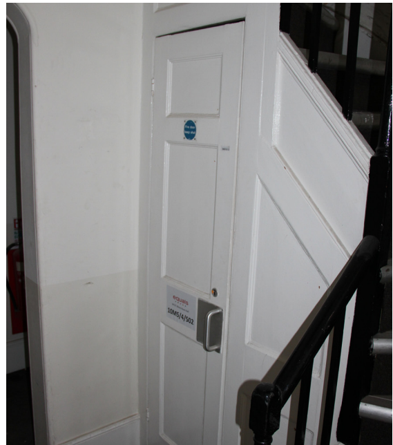
Example of existing door not suitable for fire protection upgrade. Replaced with new door to match
