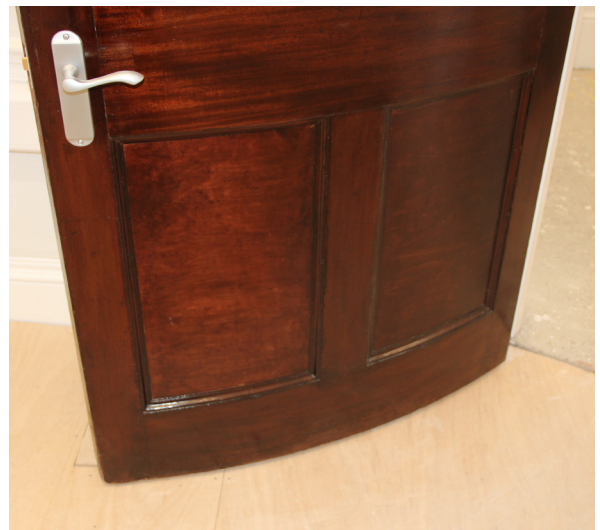
Finished door with sealmaster fireface membrane applied to curved mahogany door panels.
