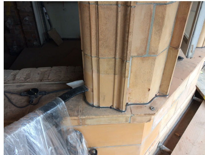
New Terracotta Tile Repair to window Surround
