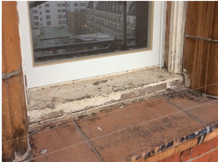
Re-pointing and Window repair/decoration
