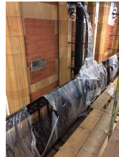
Cleaned, repaired, repainted and protected cast iron balustrade
