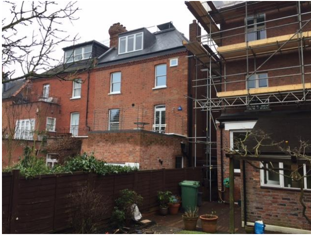
Photo 3: Rear elevation of Nos. 12, 10 and 8 Nassington Road
