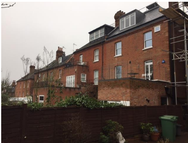
Photo 4: Rear elevations of Nos. 20 (far left) to 10 (far right) Nassington Road
