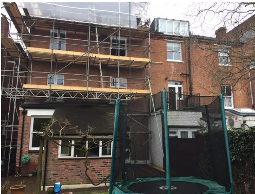
Photo 2: Rear elevation of Nos. 8 and 6 Nassington Road
