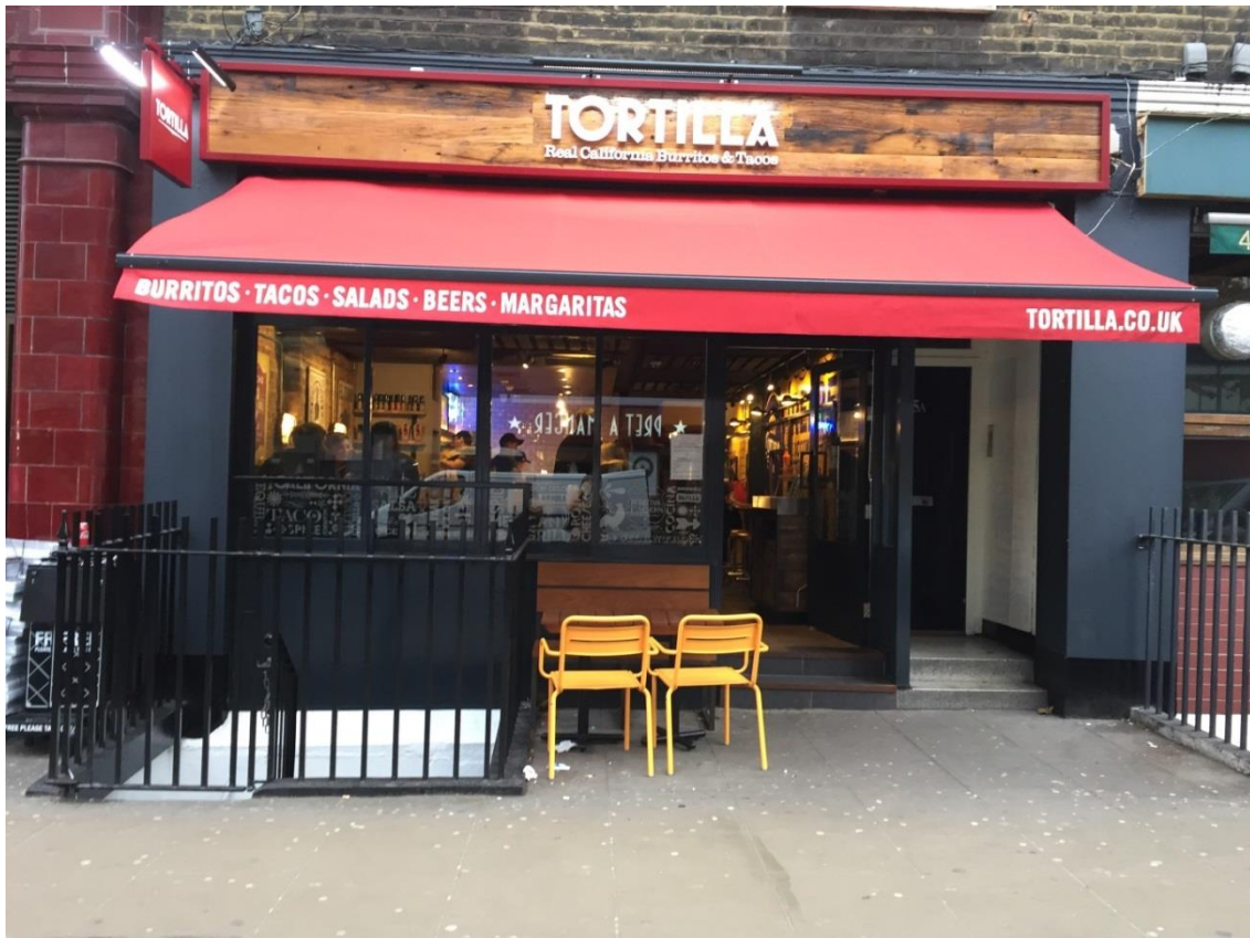
Photo 8 New Shopfront at No. 5
