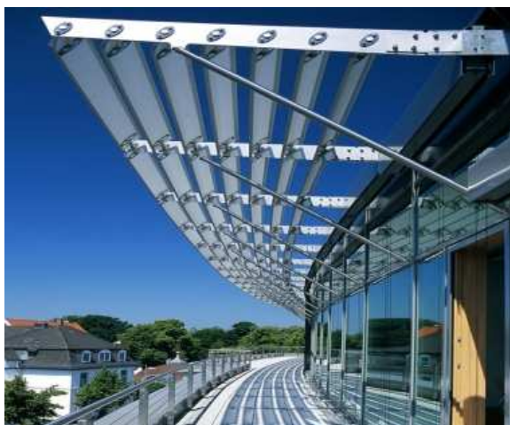
Figure 4. Solar PV Louvres on the South Facade
