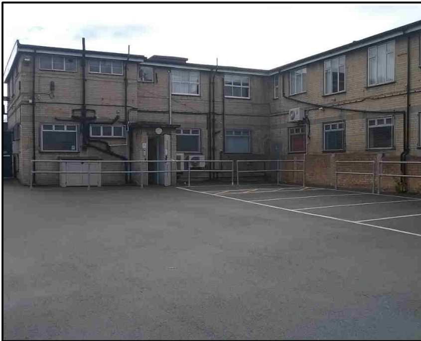
Plate 3: example of hardstanding on site looking south towards B1
