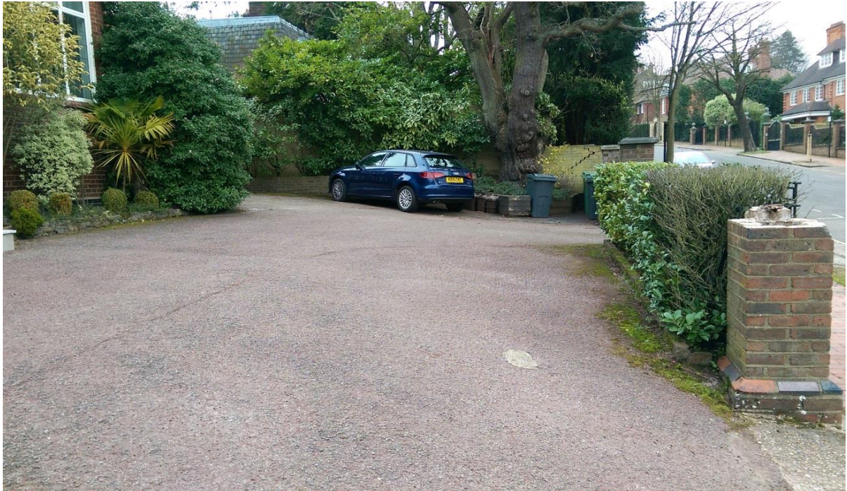
Photo 3: Externally there is a large parking/amenity area at the front of the house which is predominantly surfaced with asphalt, with a distinct fall towards the Templewood Avenue carriageway, away from the front of the house.
