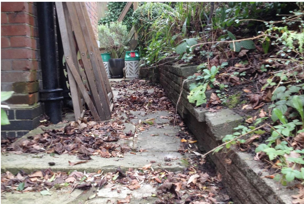
Photo 6: Immediately to the rear of the single storey extension, the low retaining wall which separates part of the rear patio from the herbaceous border was seen to be failing. It was both leaning towards the rear of the house and had slid forwards on one of the mortar beds.
