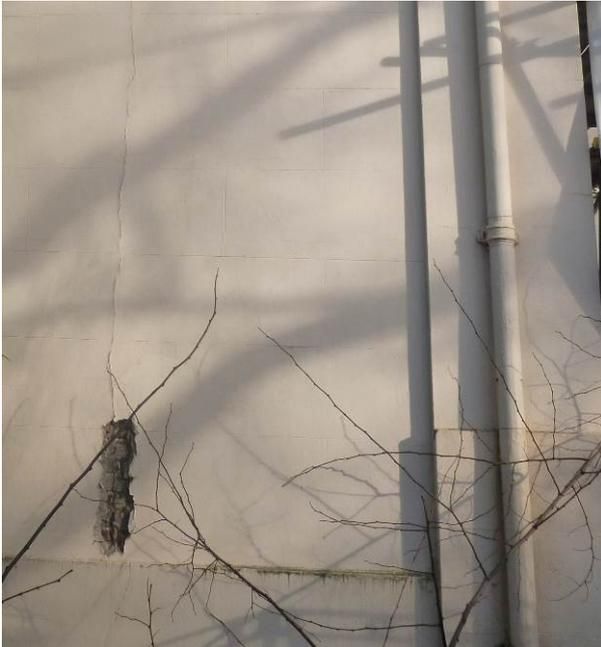
*Structural crack running full height of the building.*
