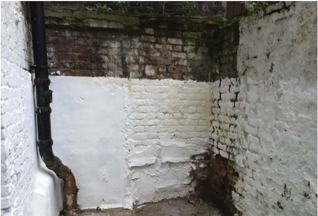
fig 6. view into existing rear courtyard
