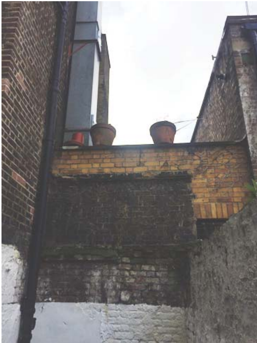
fig 5. view from existing rear courtyard
