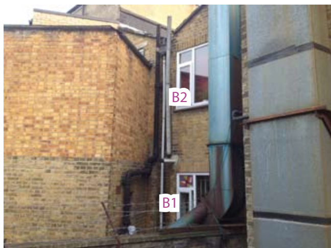
Assessed windows at 143 Queens Crescent
