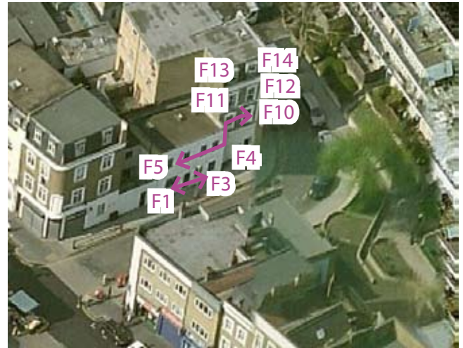
Assessed windows at Gilden Crescent
