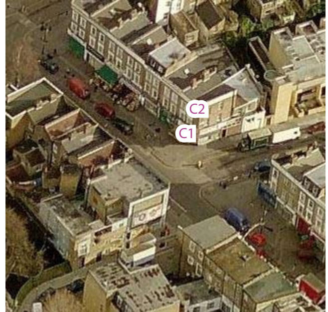
Assessed windows at 74 Queens Crescent
