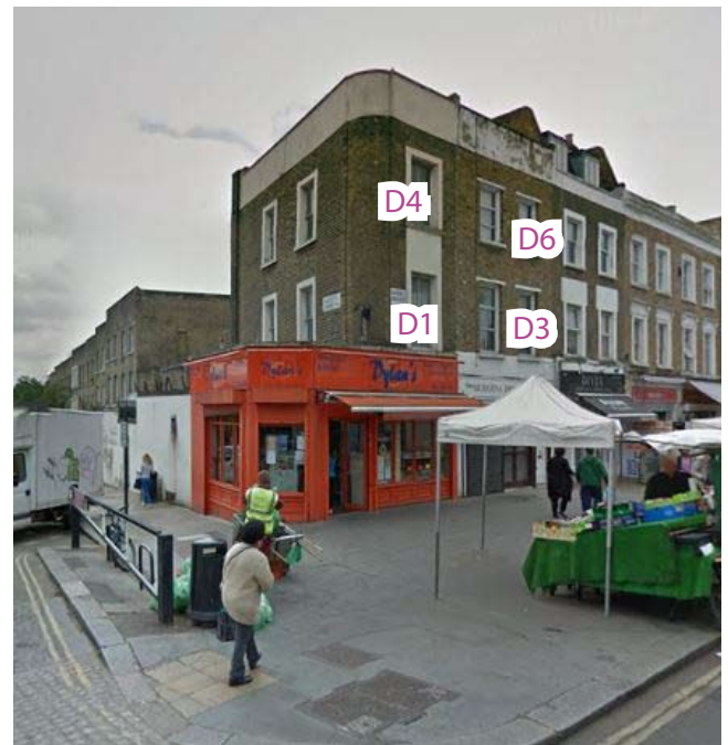
Assessed windows at 72 Queens Crescent
