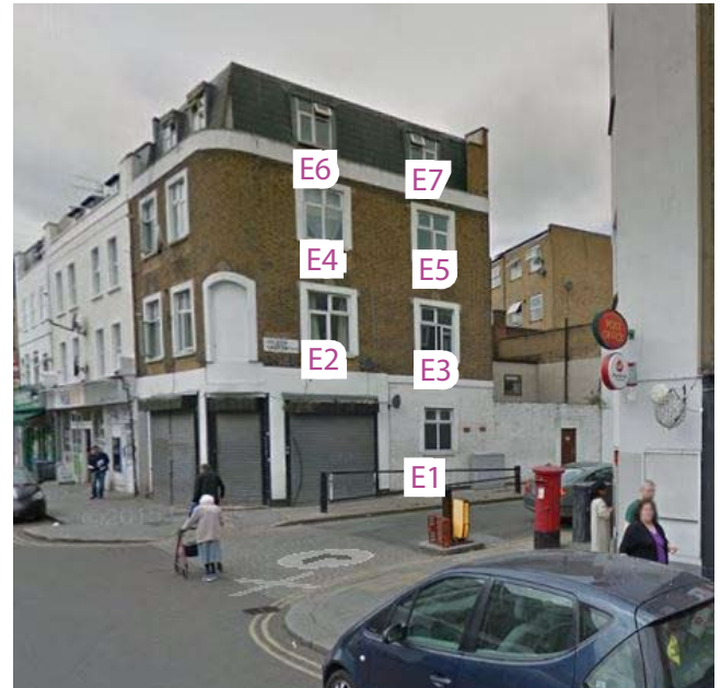
Assessed windows at 133-135 Queens Crescent
