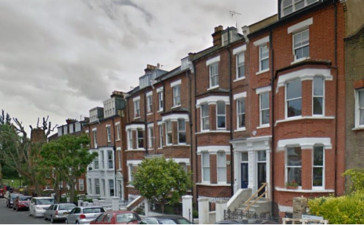
View up Pilgrim's Lane (showing front elevations)
