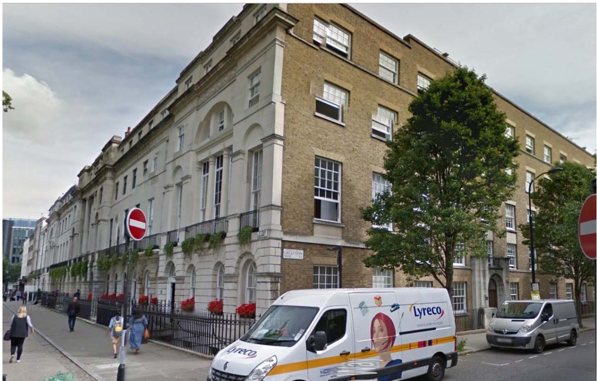
View to Adam House from Fitzroy Square
