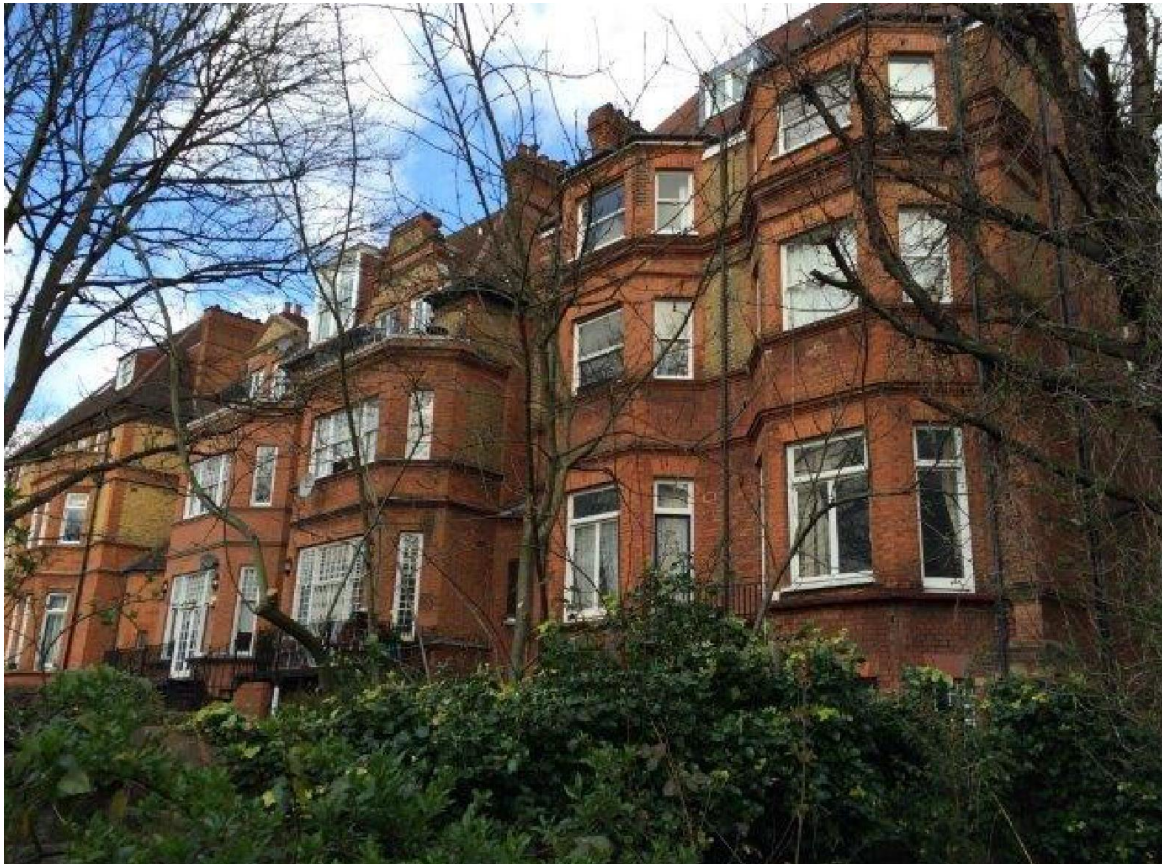
1. Rear elevation (47 Eton Avenue)
