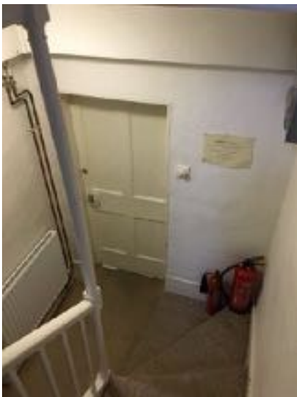
stair down to lower ground floor
