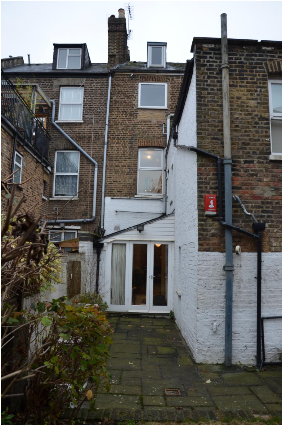
Rear of Flat 1, 8 Mansfield Road, NW3 2HN.
