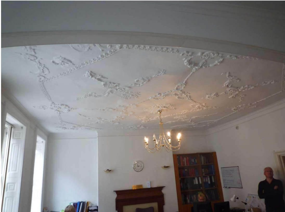
Fig. 37 Ceiling in first floor front room, from the south (AHP)
