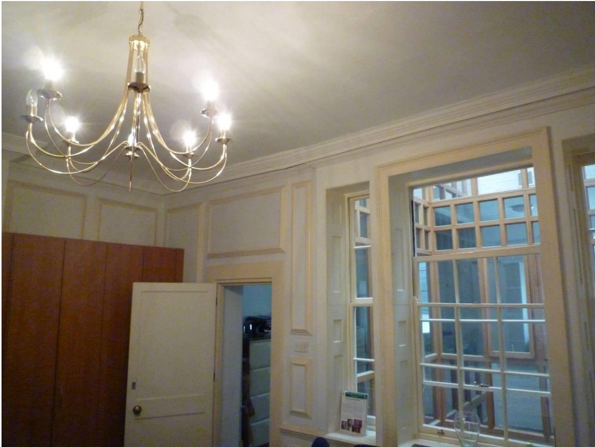
Fig.35 Panelling in the first floor rear room
