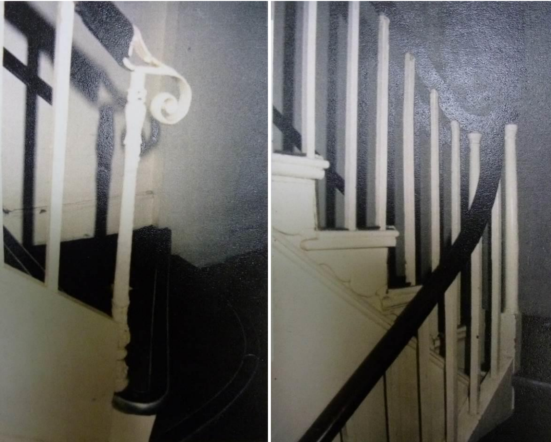
Fig. 33 Record photos of staircase, 1990 (left: ground floor newel post, right: landing between ground and first floors) (LB Camden, planning file)
