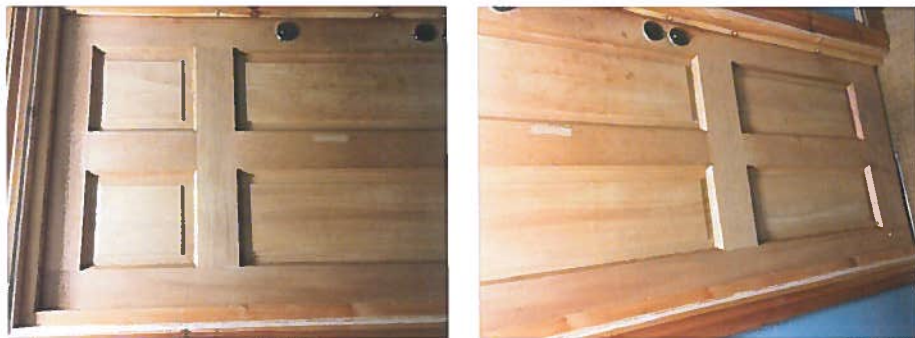
IMAGES OF DOOR AT NEIGHBOURING DOOR DETAIL
