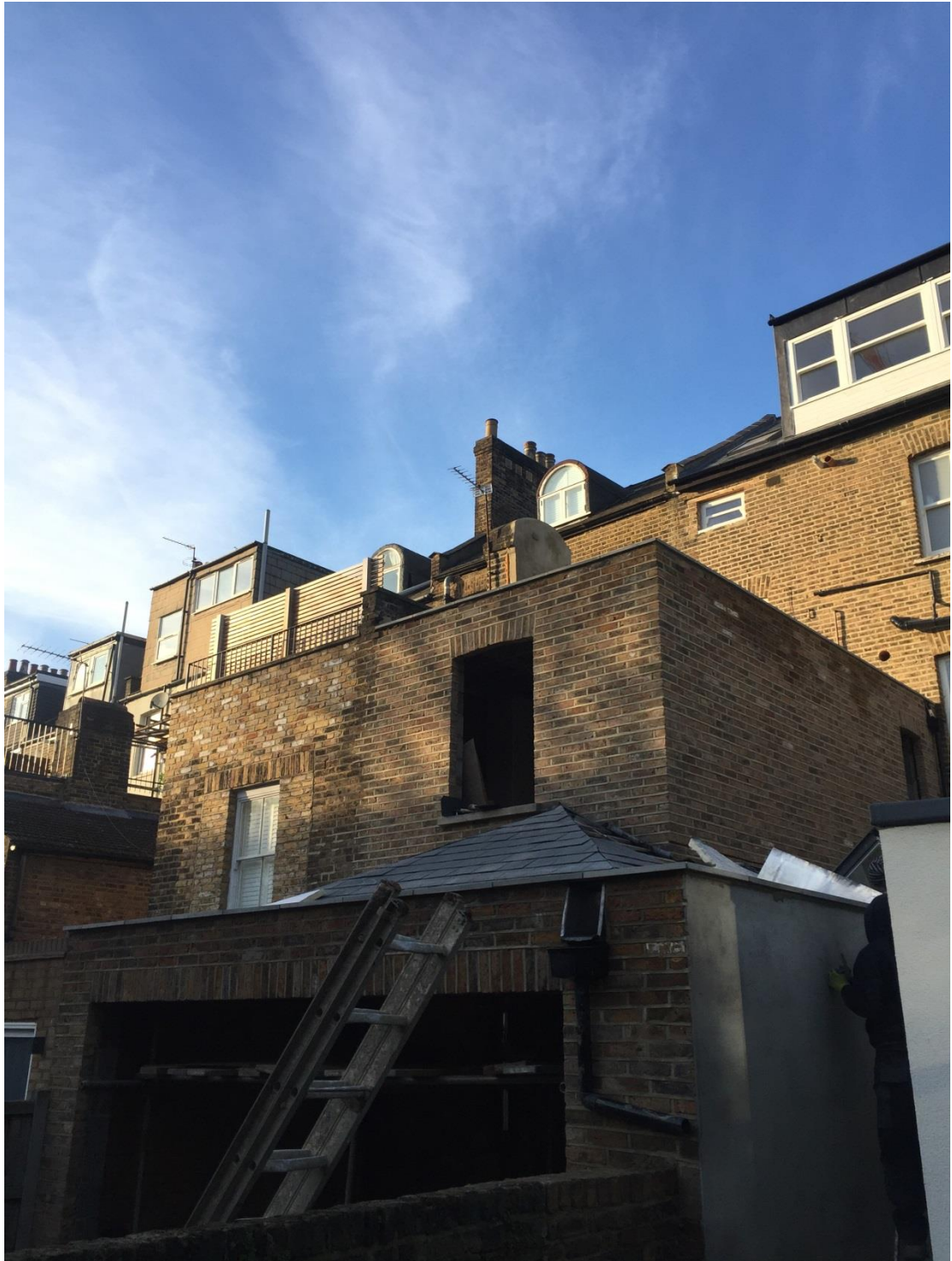
Figure 2 – View to the west of application site.
