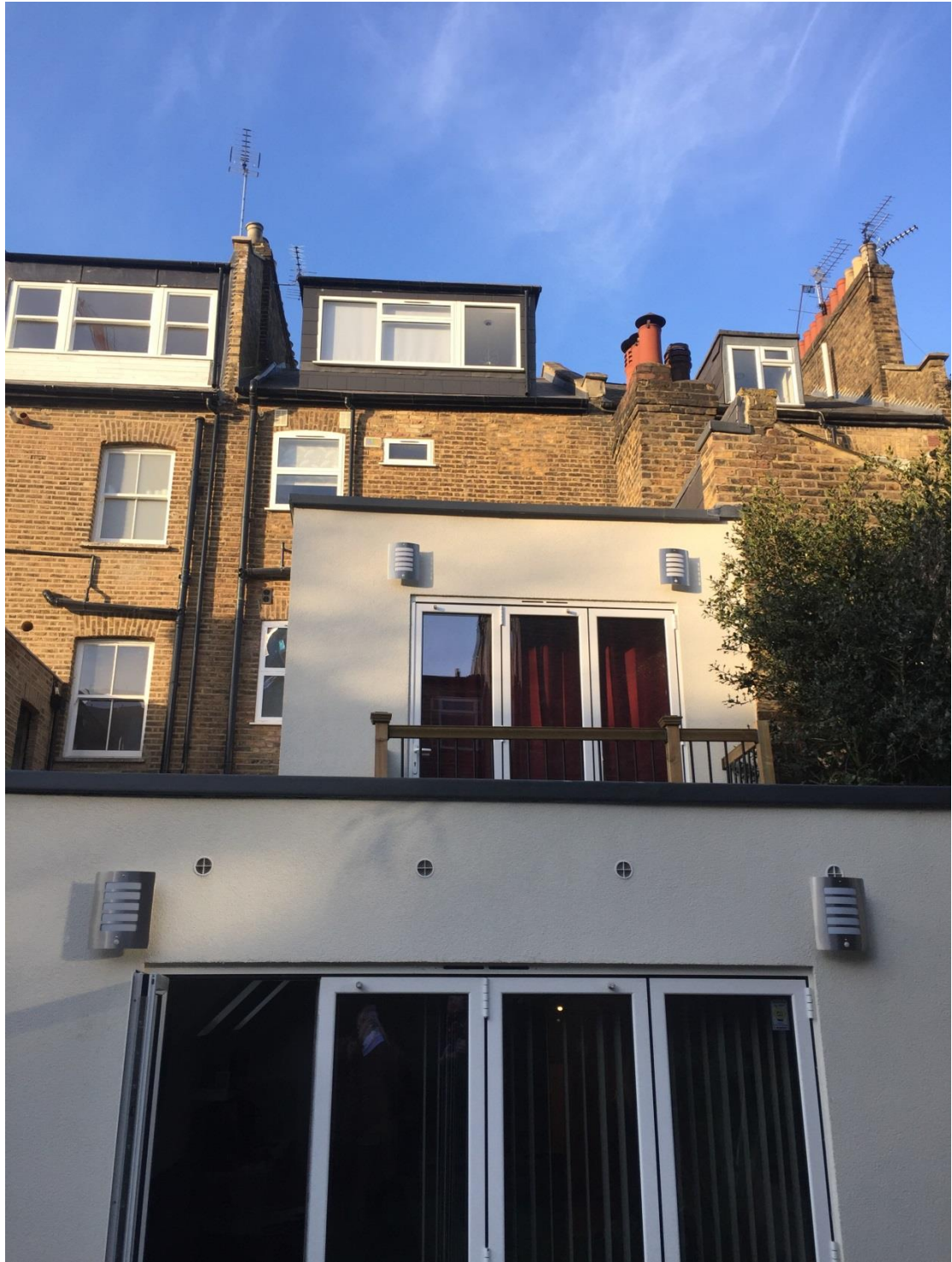
Figure 1 – Existing Rear Elevation
