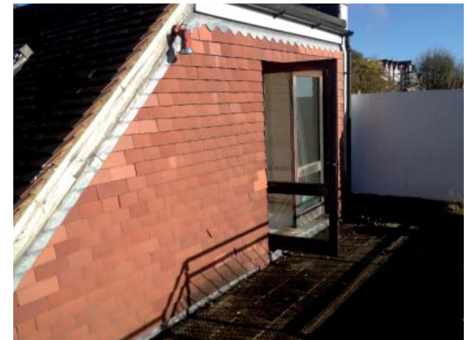
Image of existing roof access from loft
