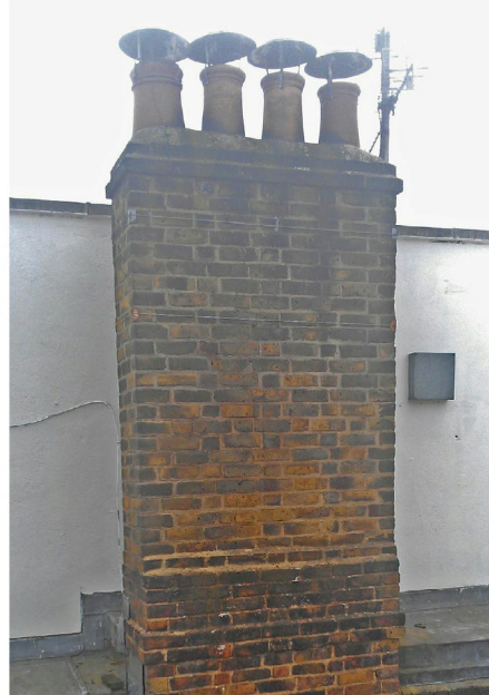
fig 8. Chimney stack extended by works at No. 36
