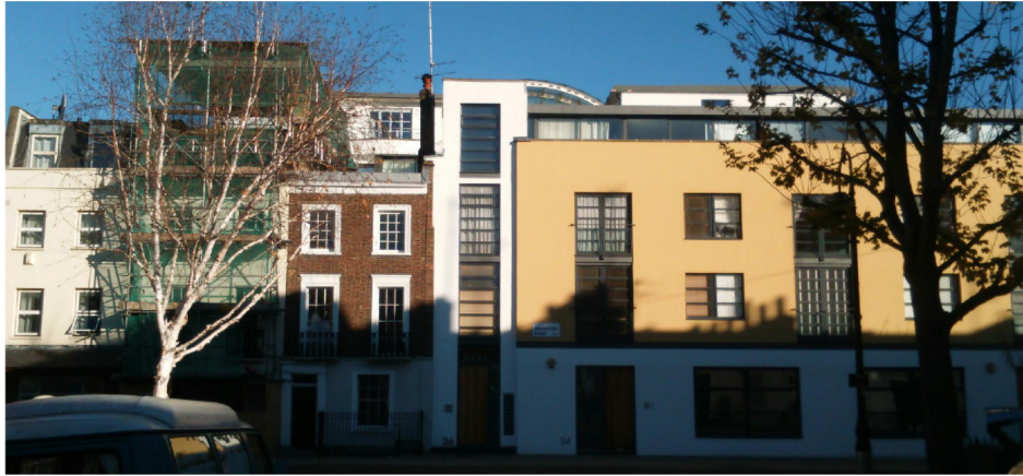
fig 1. 38 Arlington Road + Streetscape
