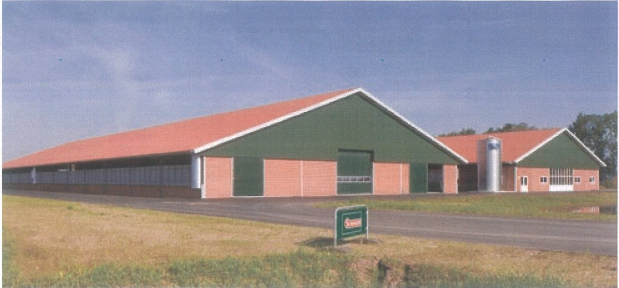
Berghorst Farm Shed, Dronten, Netherlands
