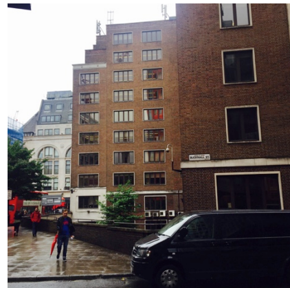
Fig.02: Building rear extending towards Bucknall Street
