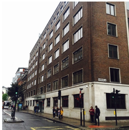
Fig.01: Building frontage (north-western corner)
