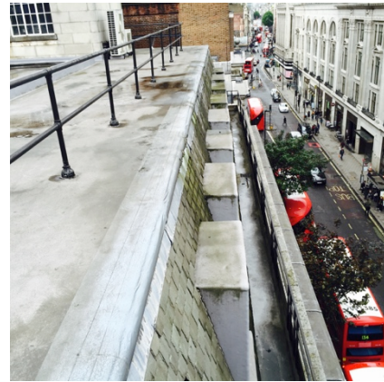
Fig.04: Roof edge overlooking New Oxford Street
