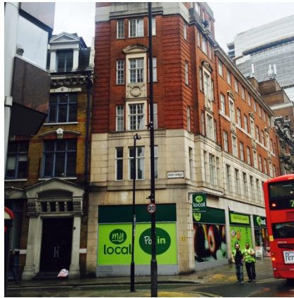
Fig.03: Building frontage (north-eastern corner)
