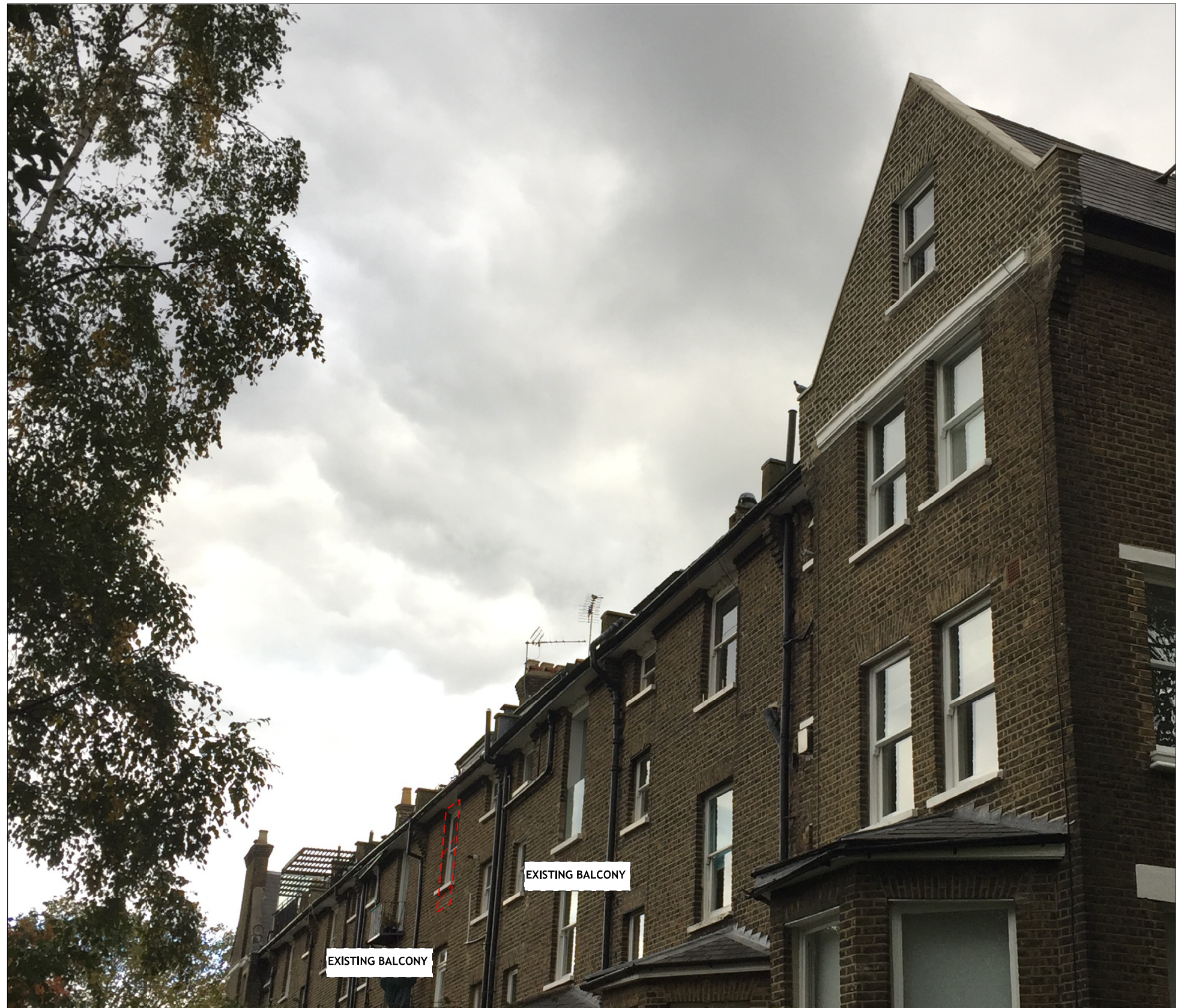
VIEW OF REAR FACADE FROM PRIMROSE HILL PARK
