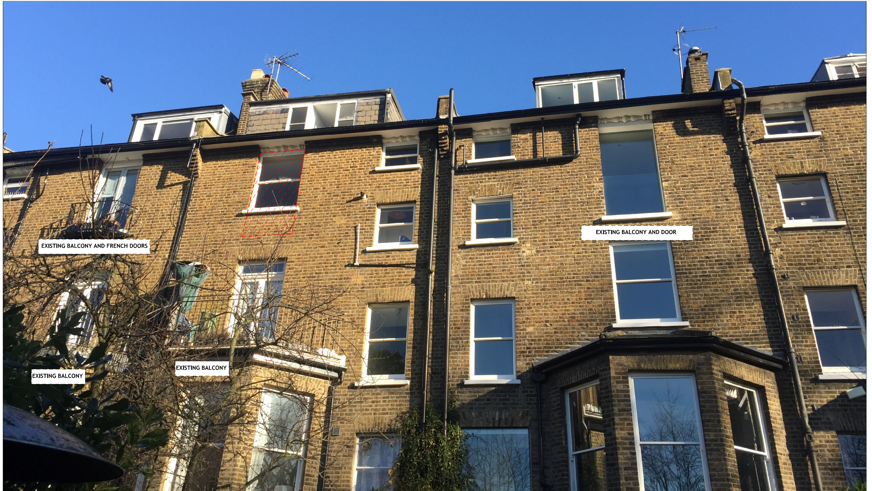
WEST FACADE - REAR ELEVATION
