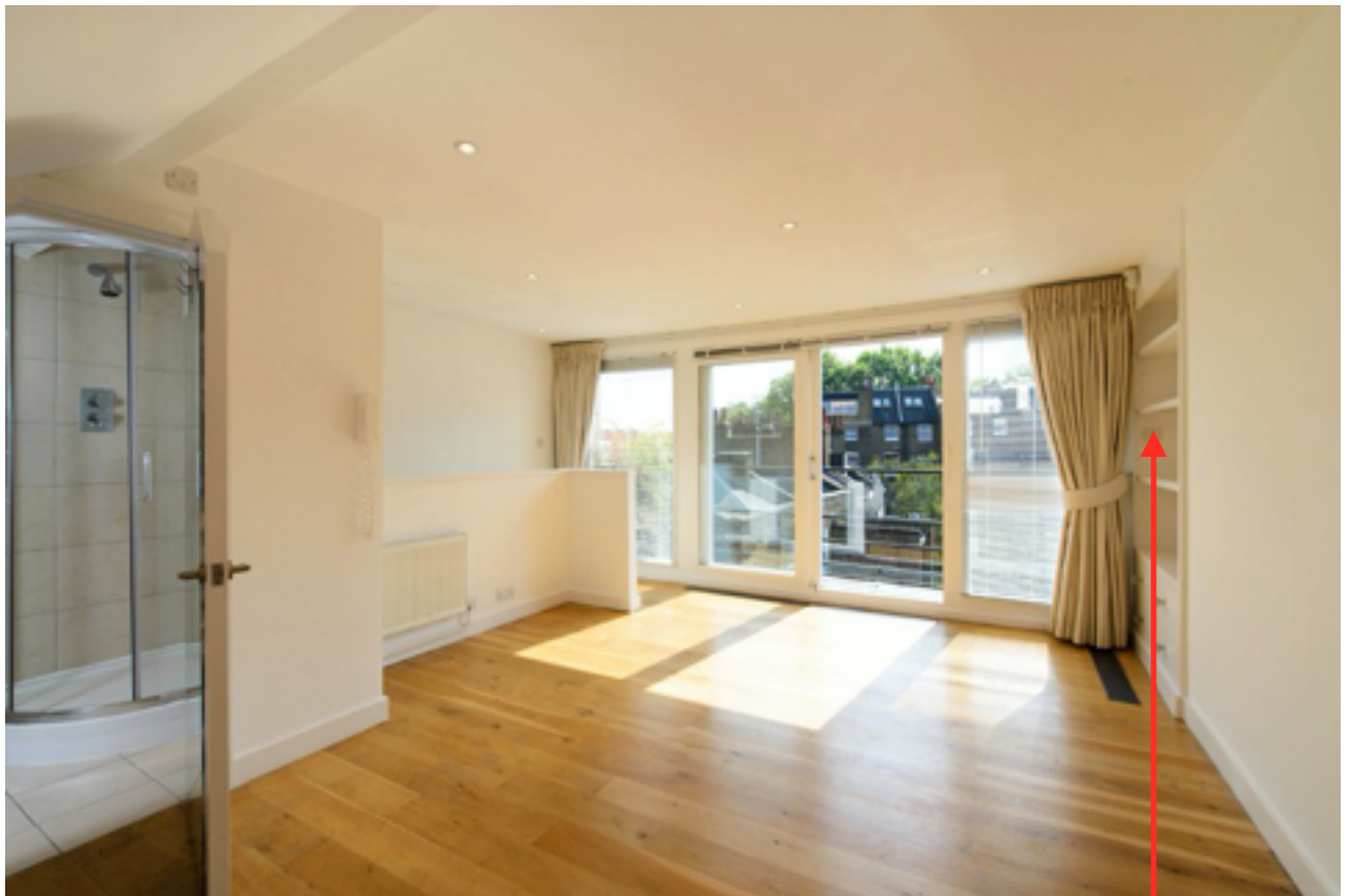
Photograph of third floor bedroom - AC unit will sit within this recess.
