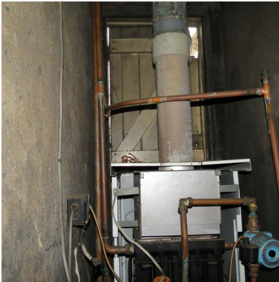
fig 7 & 8. Asbestos containing boiler + kitchen in need of modernisation
