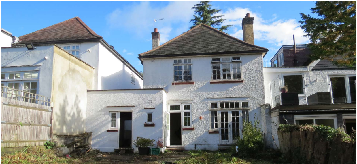
fig 2. 89 Hillway - rear elevation
