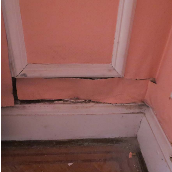
fig 5 & 6. Internal damage caused by damp, ground floor
