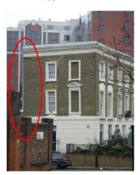
The report suggests that one contributory factor to the lean may be the 'butterfly roof' construction, exerting pressure on the end wall as shown in this illustrative diagram:
