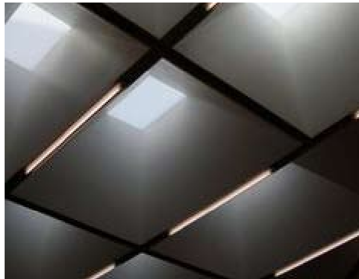
Coffered ceiling with rooflights
