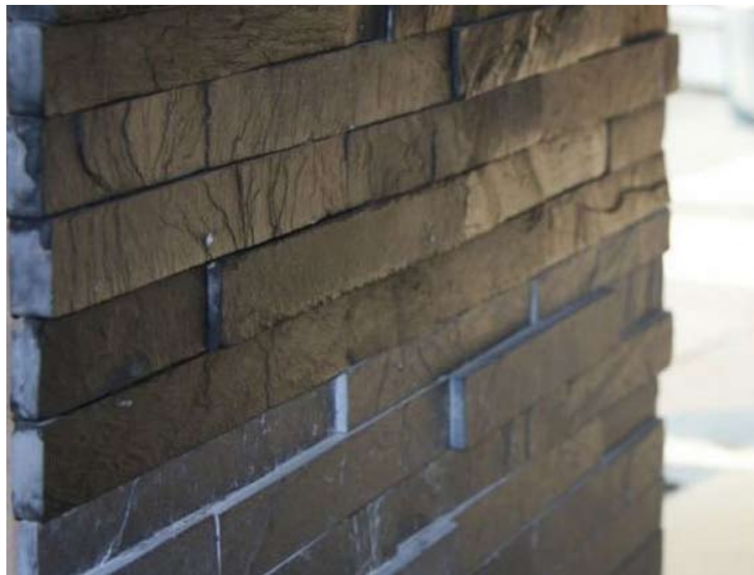
Black basalt cladding to walls
