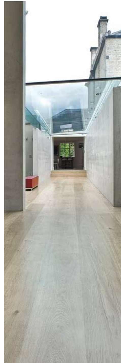
Douglas fir flooring/decking running from inside to outside
