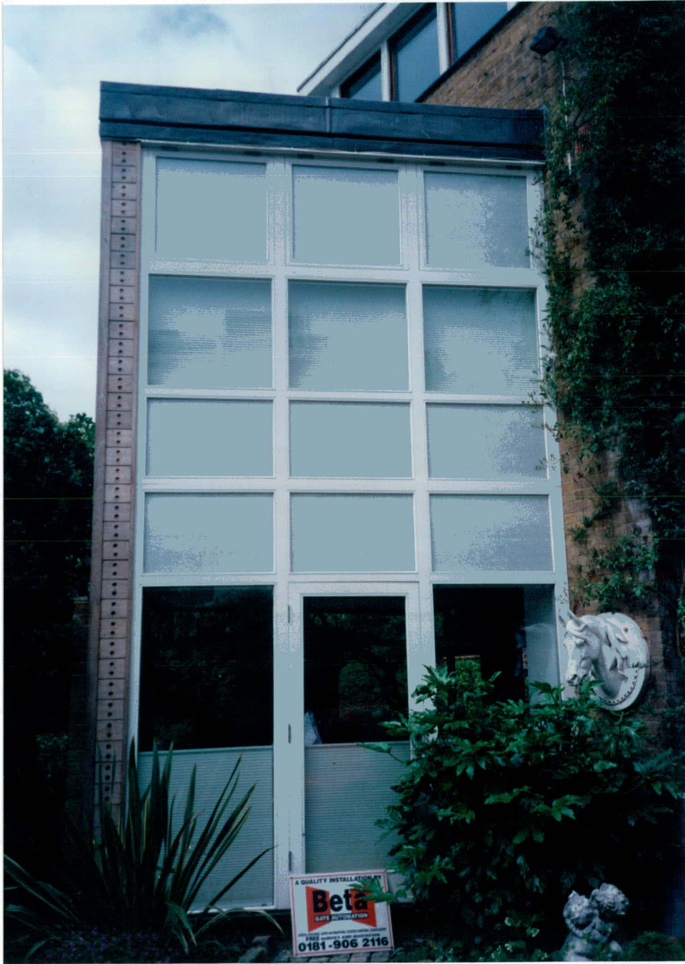
EXISTING KITCHEN AND BEDROOM EXTENSION SHOWING THE USE OF OKALUX
