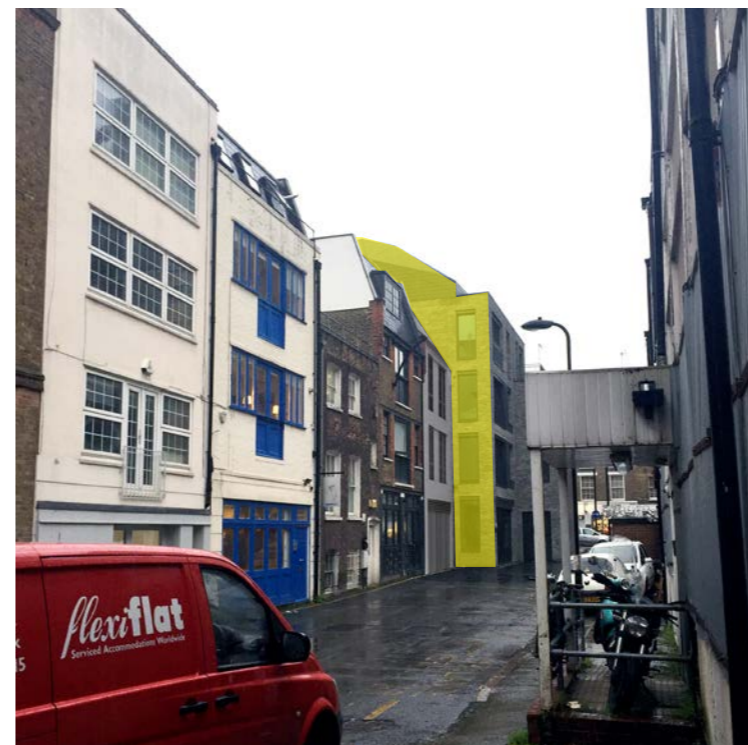
Consented Scheme: The flank wall is partially covered. The roof extensions is still in full view.
