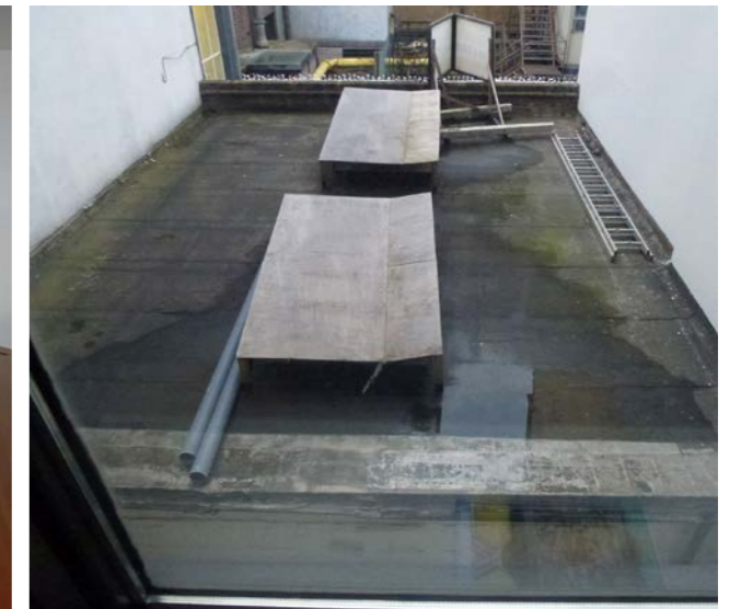
View from First floor window, looking south
