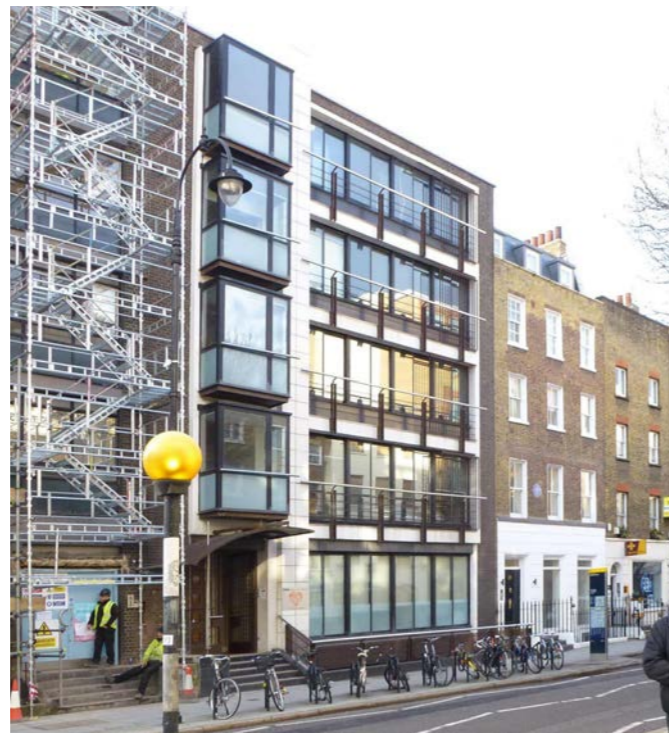
Existing Building front elevation
