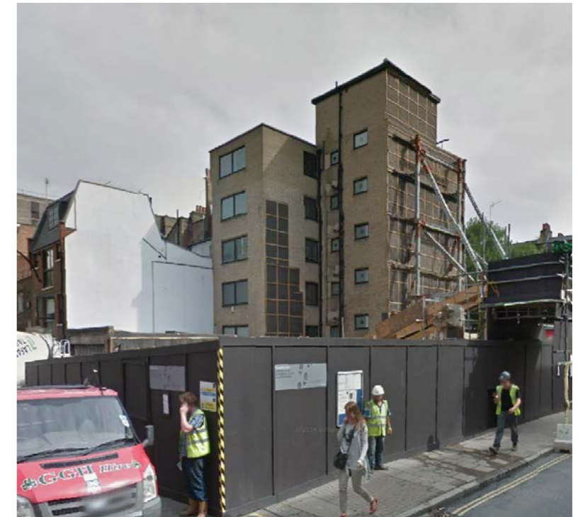
Currently exposed side and rear elevations
