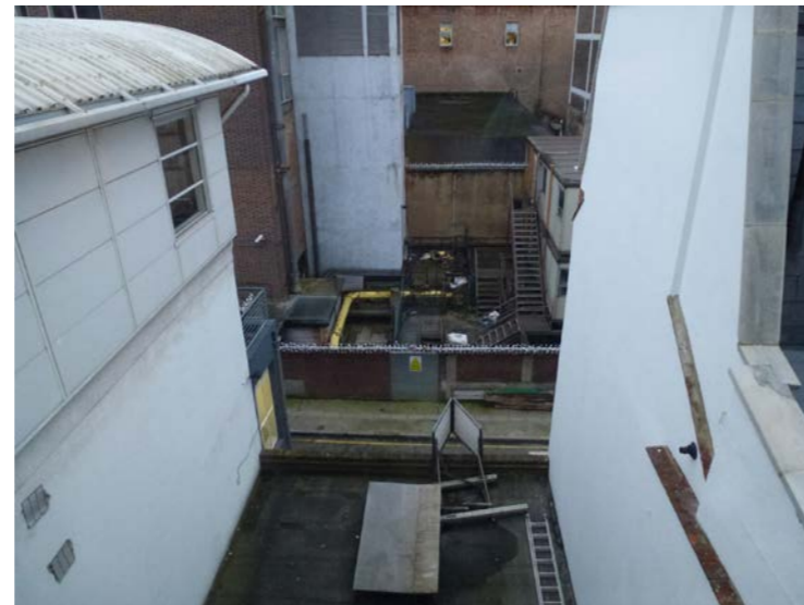
View from First floor window, looking south
