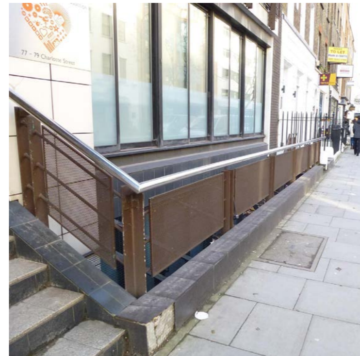
Existing Building - inactive frontage
