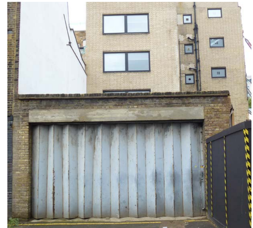
Existing Building rear elevation
