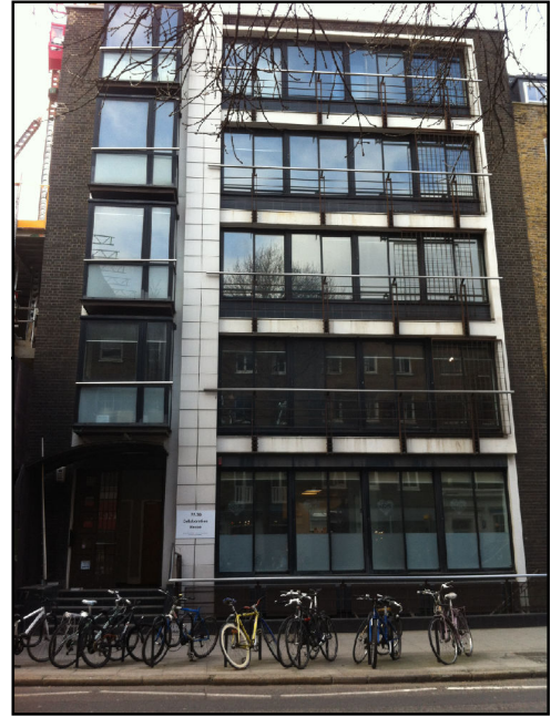
Photograph 2: Existing building (B1 on Figure 2).
