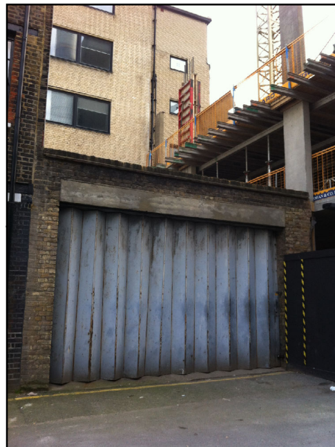
Photograph 3: Garage onto Tottenham Mews (B2 on Figure 2).
