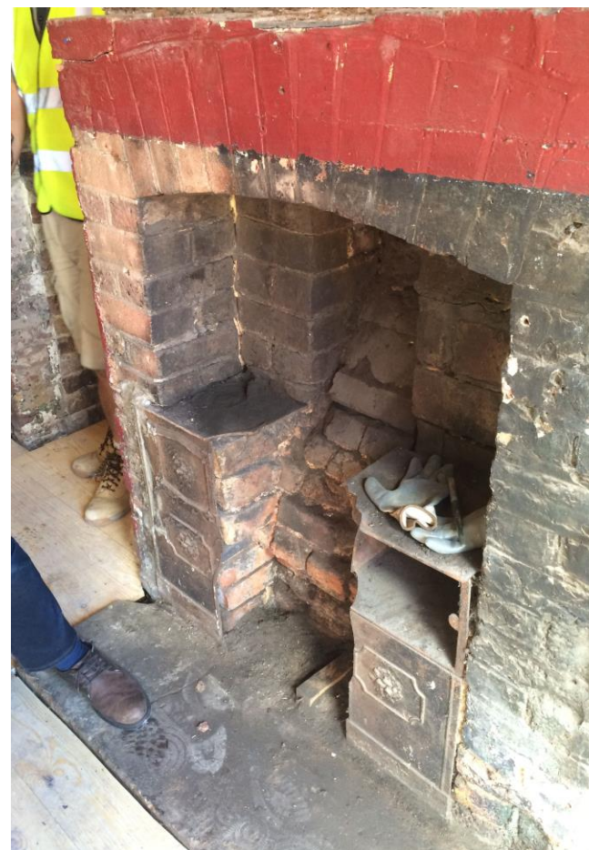
Figure 8: Chalk Farm Building, ground floor: north room fireplace showing fragmentary cast iron hob grate (unit 39).
