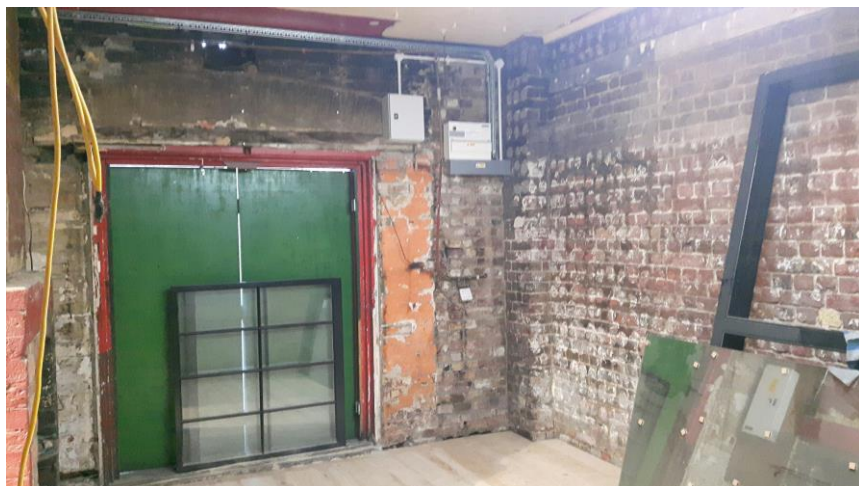
Figure 7: Chalk Farm Building, ground floor: view within north room (unit 39).
